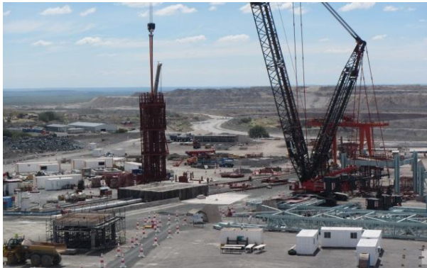
Venetia Underground shaft sinking
